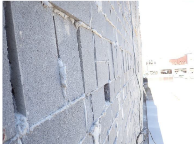
Figure 2. CMU infill outboard of steel spandrel.
