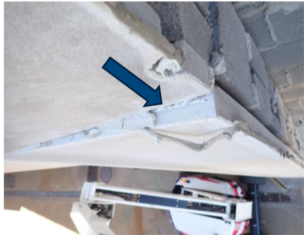
Figure 6. Impacted and rotated stone panel.
