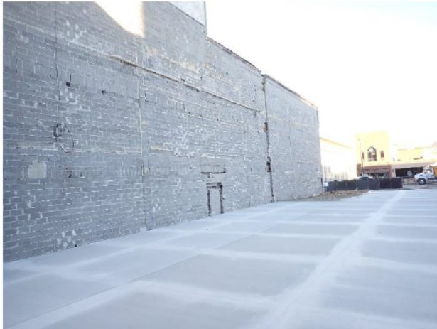
Figure 1. Overview of north end of east elevation.
